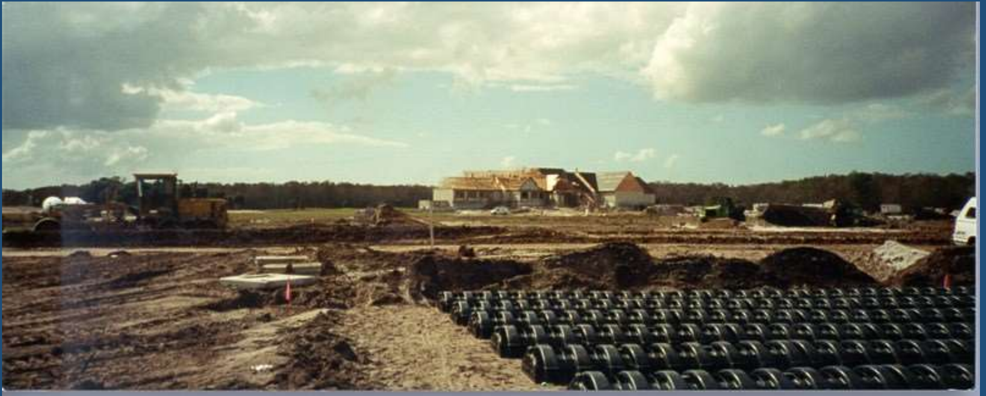
Dispersal System located in a central area
